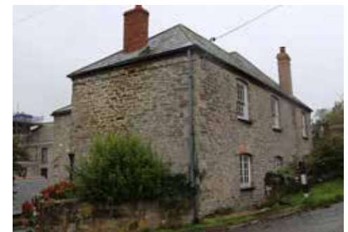
Figure 47: Space for green infrastructure. Example shows how rain garden planter could be detailed beside downpipe.
