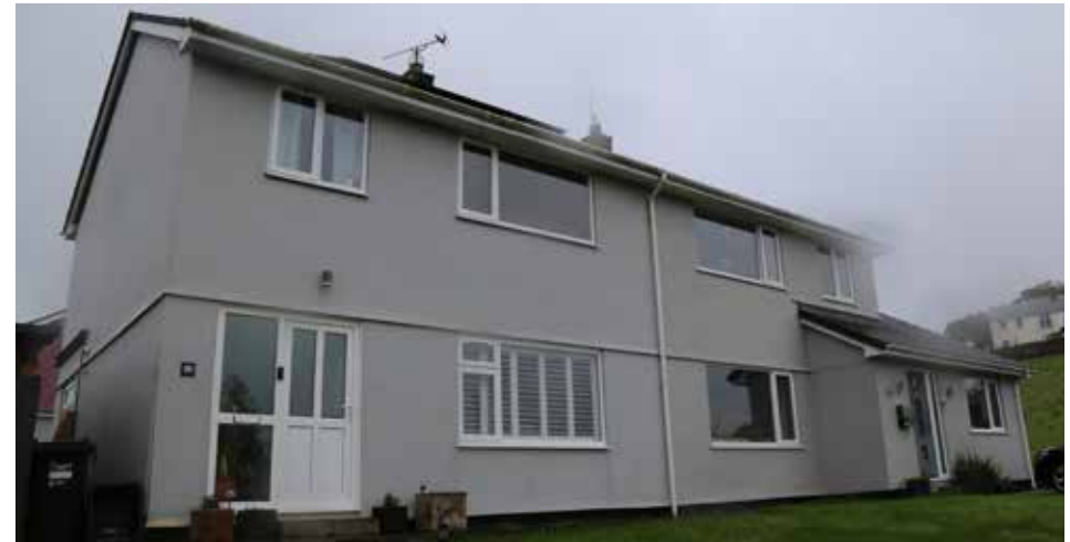
Figure 31: Development which is not reflective of Cornish settlement character.
