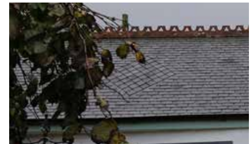
Figure 68: Slate roof, with contrasting ridge tiles.
