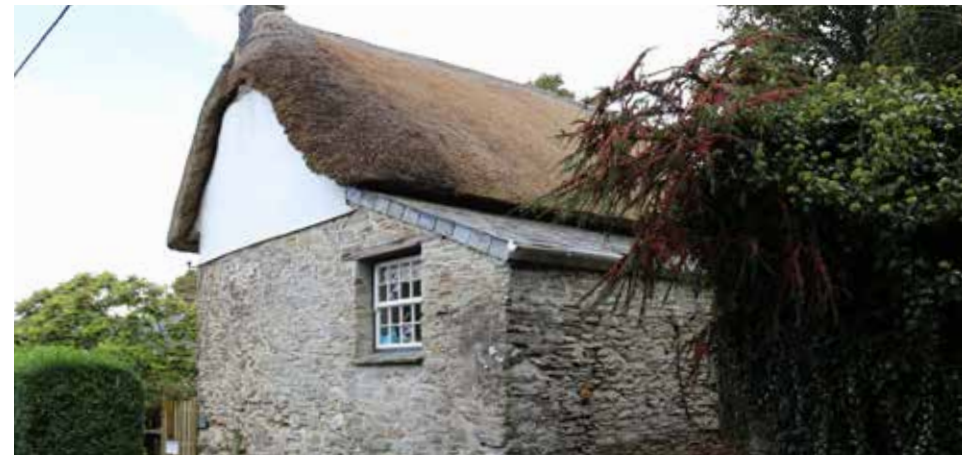
Figure 36: Distinctive traditional material usages. Stone, likely cob upper storey with thatch and slate roof.
