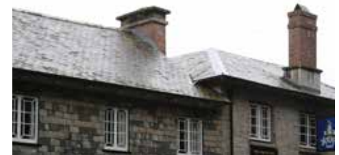
Figure 49: Roofscape variation, and red brick chimneys.
