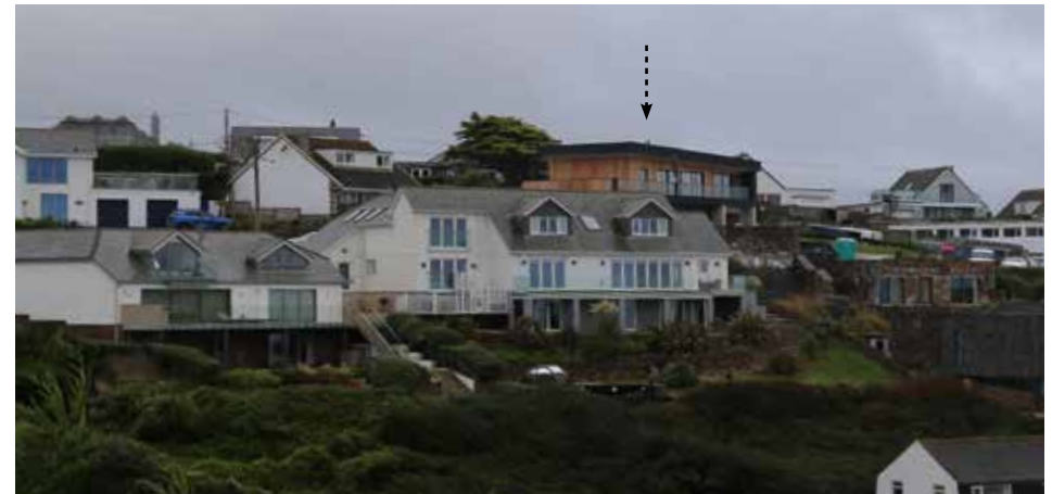
Figure 18: Example of a two and a half storey property (foreground) with renovated flat roof property behind to the same ridge height of neighbouring pitched properties.
