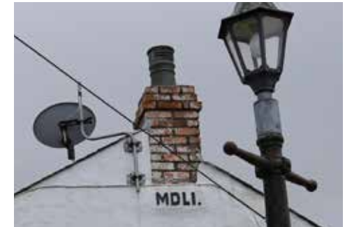
Figure 67: Red brick chimney.
