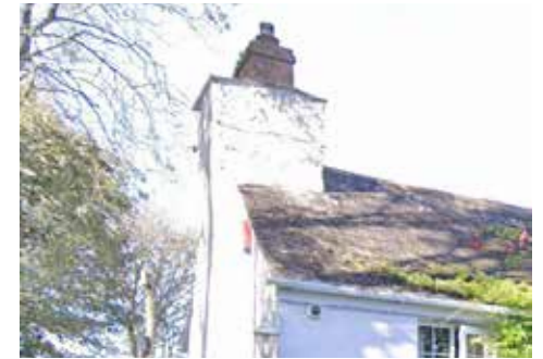
Figure 70: Gable projection chimney.
