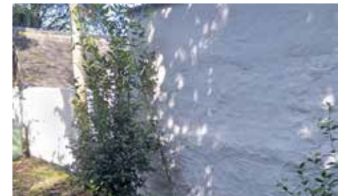
Figure 71: Lime wash finish to boundary wall.
