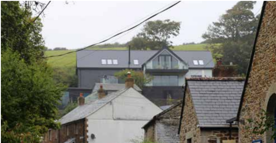
Figure 30: Overbearing and out-of-scale dwelling within the Conservation Area.
